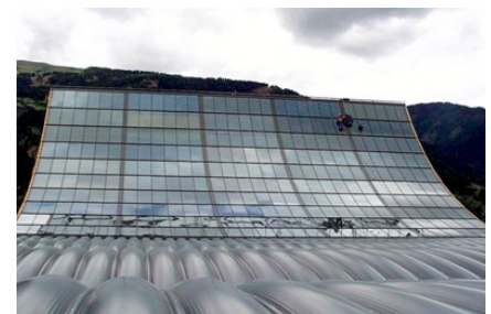
Fig. 3: Solar plant (source: Austriasolar)
